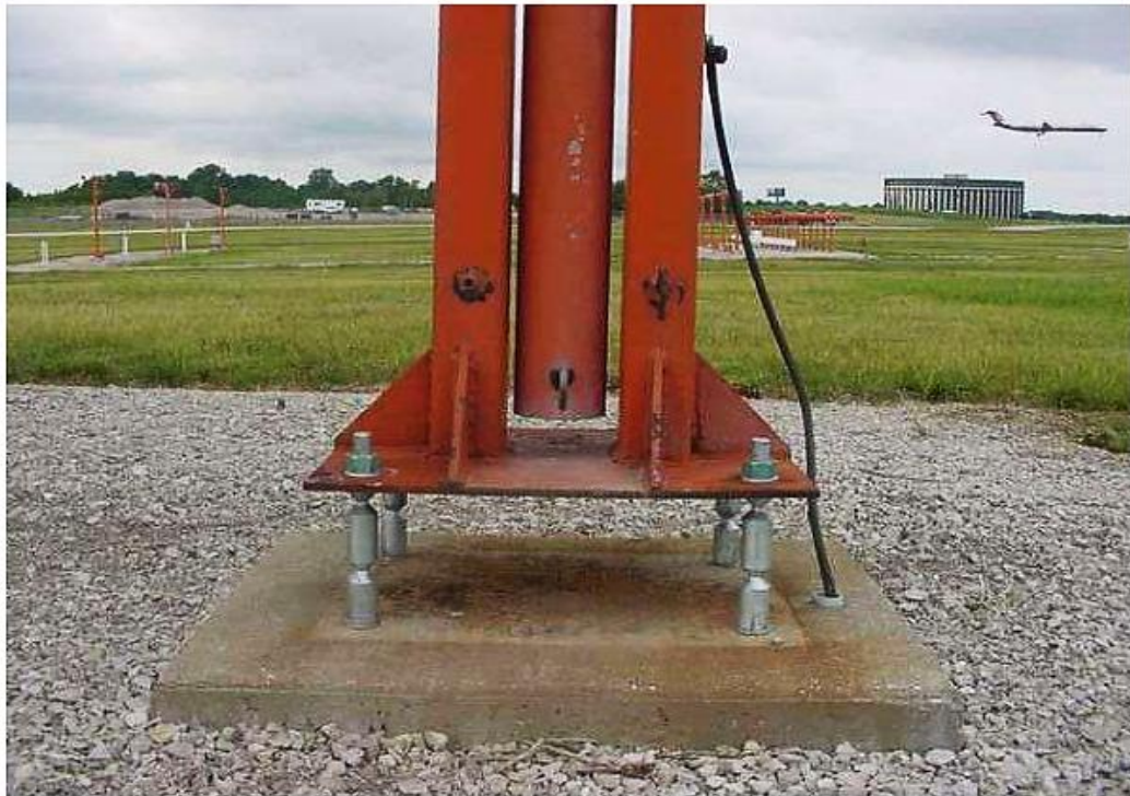
Figura 2-6-1. Perno fusible.
